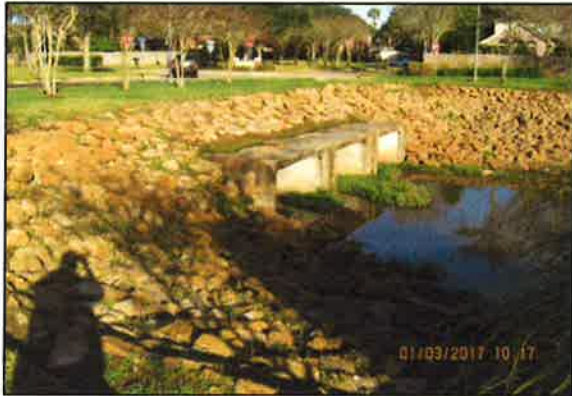
Existing Riprap (Loose Recycled Concrete)
